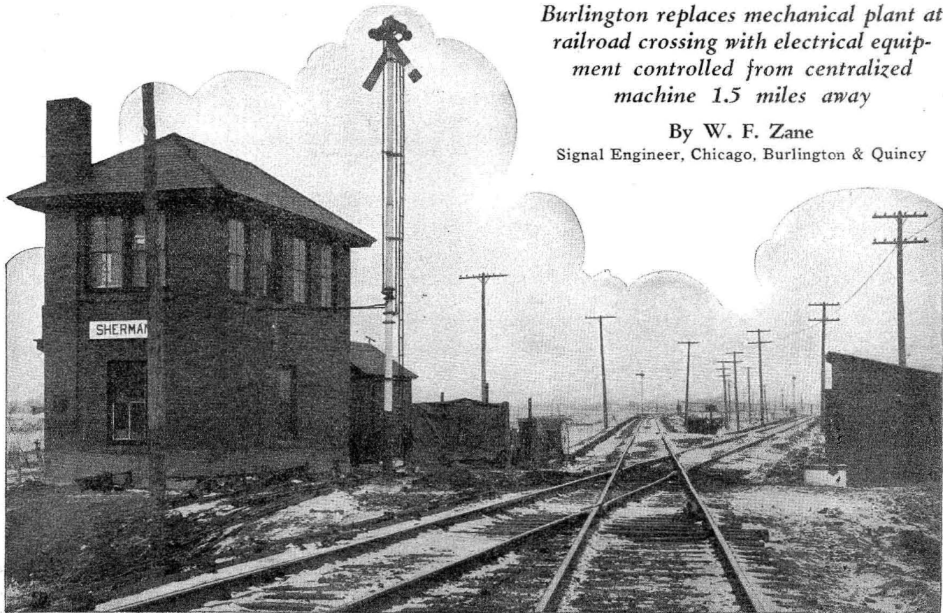
Tower building and all mechanical fittings will be removed shortly—New remote control facilities in wooden shelter at right
