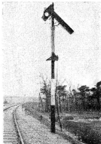
Fig. 2.—Caution signal at warning—Green light
