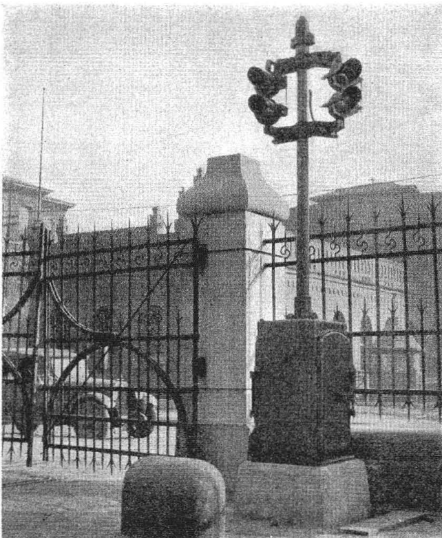
Color-light signals, designated as indicators are used for the information of the enginemen
