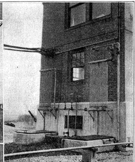
Aerial cable lead carried through wall of tower
