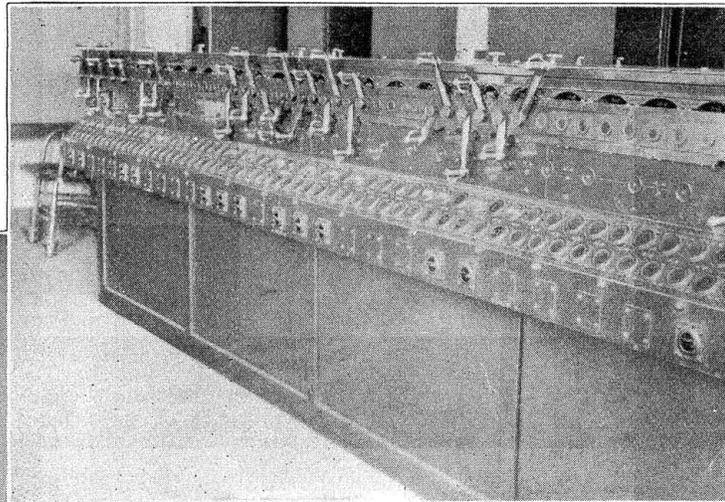
*All control wires are carried in overhead cables*
