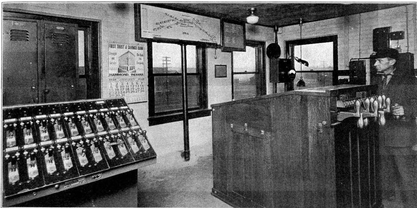
Tower operating room containing yard switch control machine (left), illuminated track diagram and electric interlocking machine (right)
