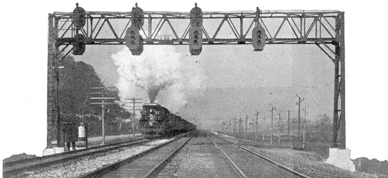
Eastbound train approaching bridge 6 at NC cabin
