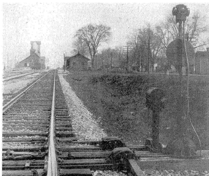
Hand Throw Switch at Chebanse With Electric Lock
