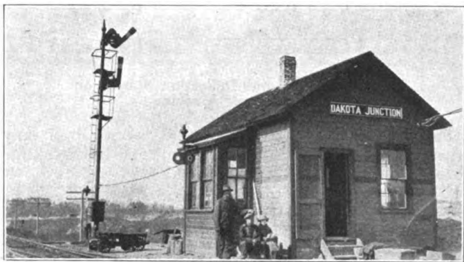
Westbound Approach Signal and Operator's Cabin
