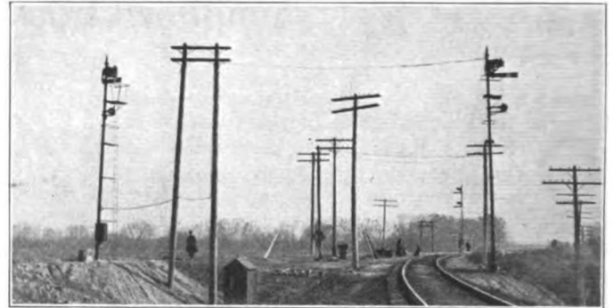
Eastbound Home Signals
