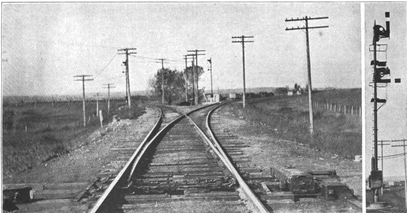
Switch Machine Layout With Eastbound Home Signals in Rear and Westbound Home Signal at the Right
