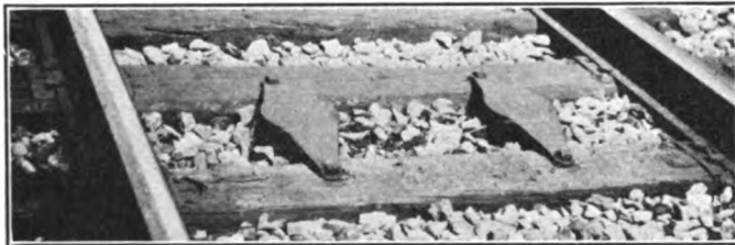
The Two Pole Pieces of a Brake Application Magnet. The Permanent Magnet Which Connects Them Is Underneath the Ballast
