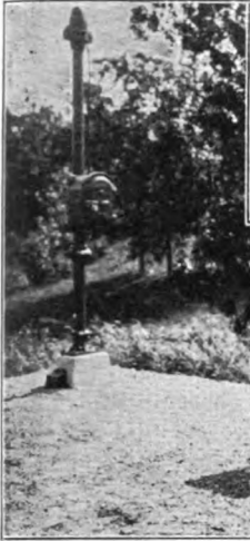
Dwarf Signal and Telephone at End of Passing Track.
