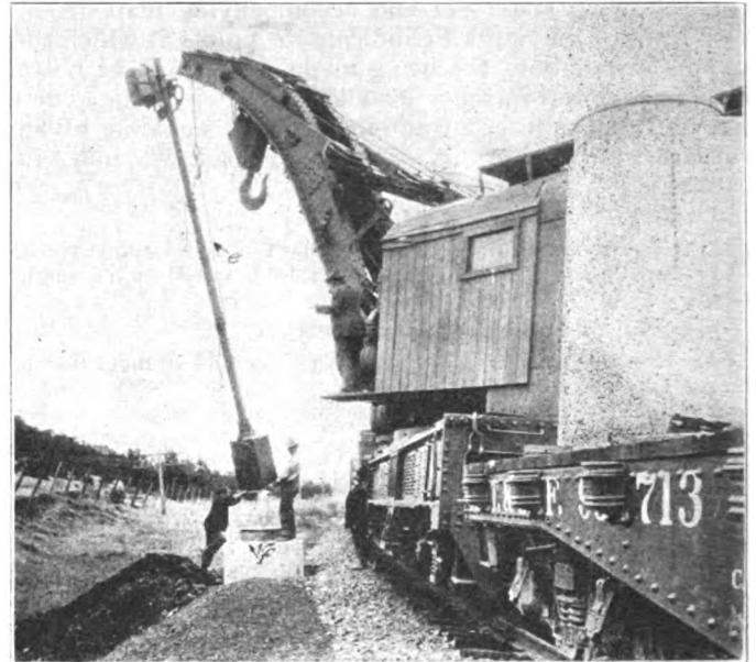
Assembled Signal, Mast and Relay Box Being Installed
