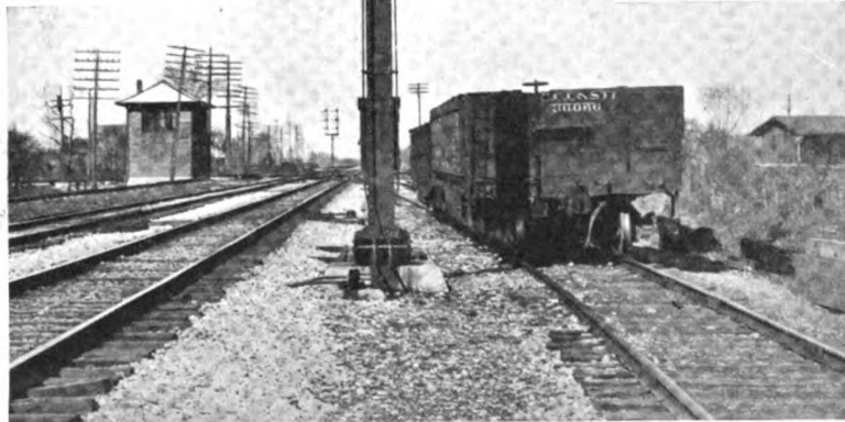
Home Signal Boyd Interlocking Two Top Arms Power Operated 221
