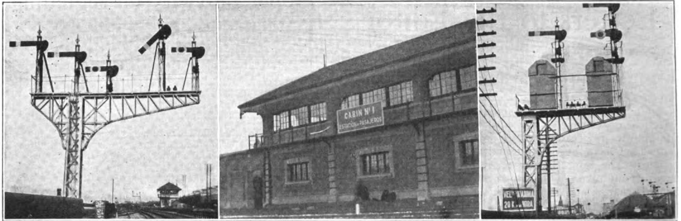
Signal Bridges and Tower, Retiro Station, Buenos Aires
