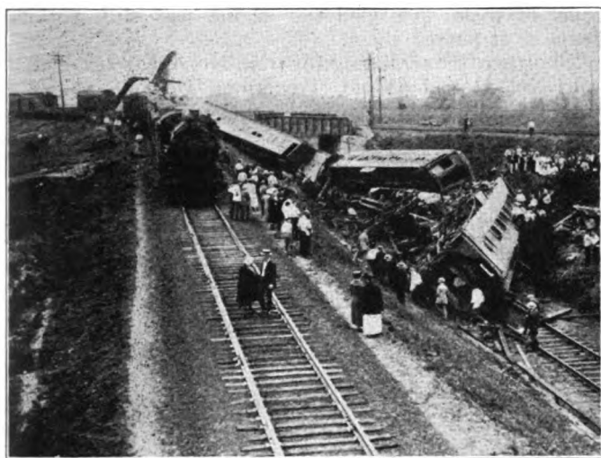
View of Wreckage on West Jersey & Seashore Tracks
