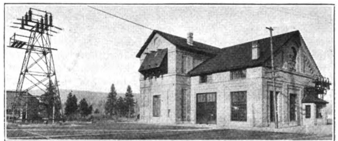
Exterior of Cle Elum Substation
