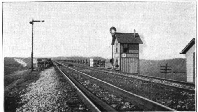
East End of Boone Bridge, Showing Old Mechanical Signal, Later Changed to Power-Operated Signal
