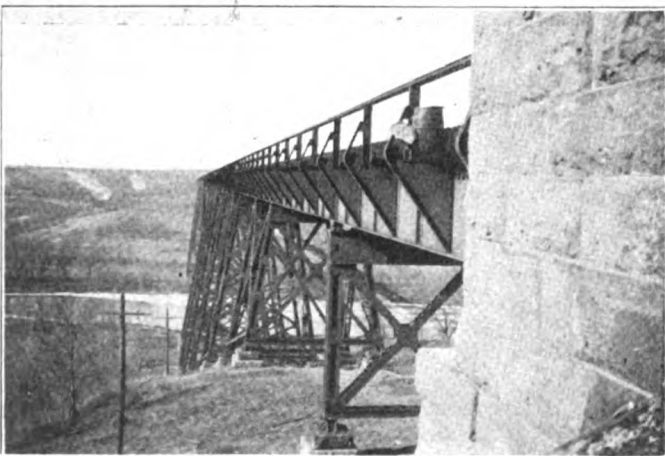
A View of Boone Bridge from the East Abutment
