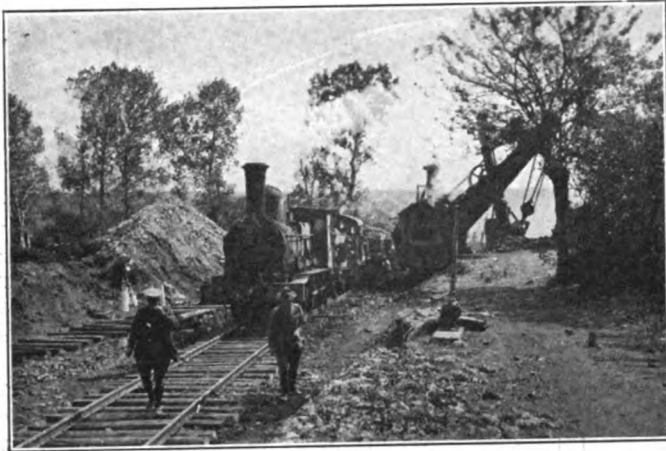
Steam Shovel Loading Dump Cars; Nevers Cut-Off
