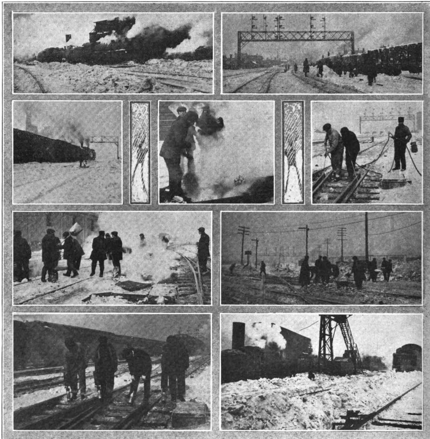
Ready for Emergencies "Double Heading" Clearing the Tracks Using the Kerosene Burners
