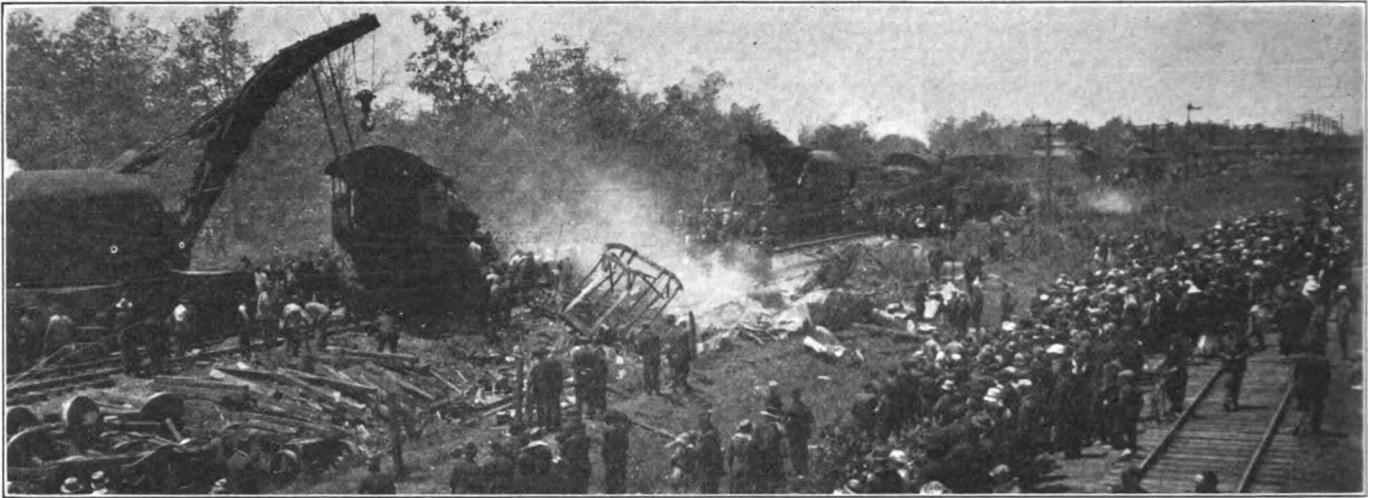
A General View at Ivanhoe, Showing the Debris, the Gary & Western at the Right and the Home Signal in the Distance
