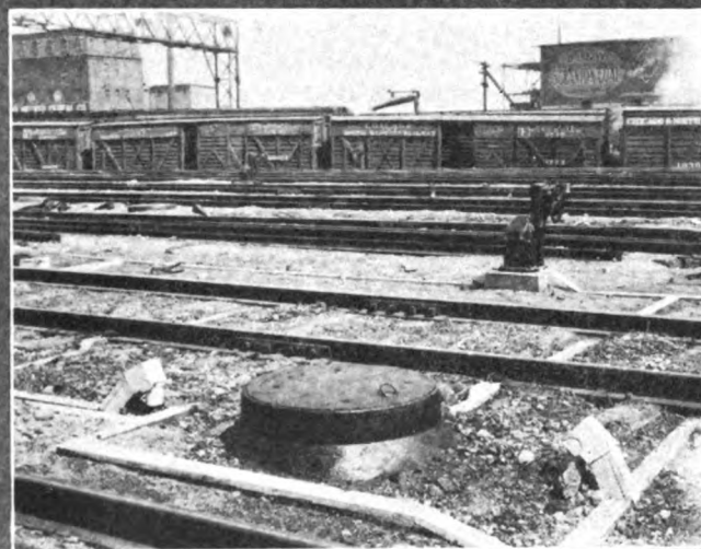
The Shop and Tower from the C. M. & St. P. Tracks The Three Northbound Home Signal Bridges Trunking Runs, Special Caps, and a Dwarf Signal
