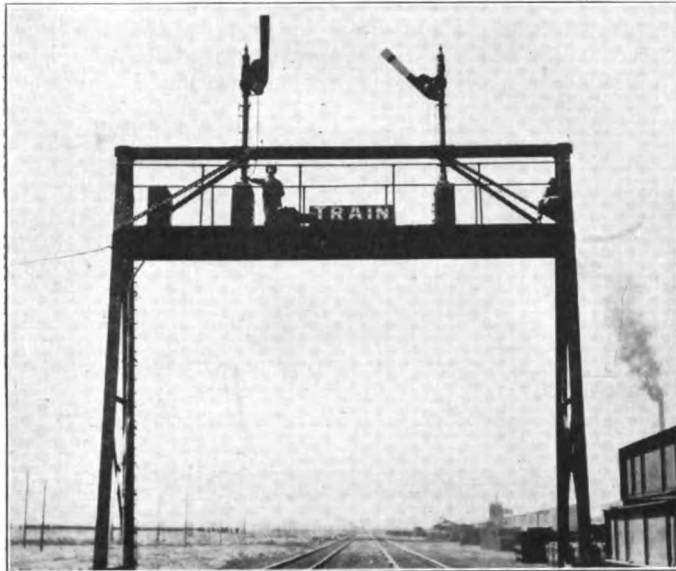
One of the Train Signs Mounted on a Signal Bridge.
