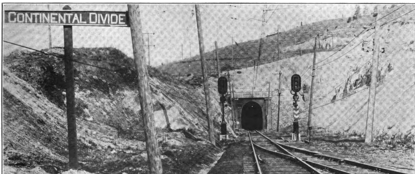
Double Location at Portal of Tunnel on the Summit of the Rockies.
