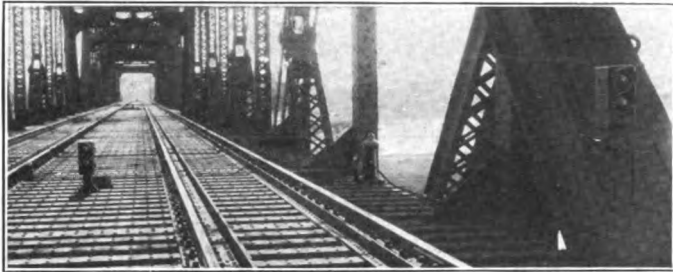
Looking East Over the Draw Span Showing Two Dwarf Signals and Track Instrument.
