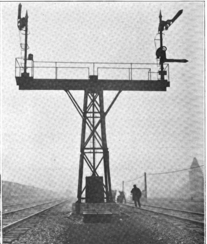
The Double Cantilever Bridge Supporting the Eastbound Distant Signal.
