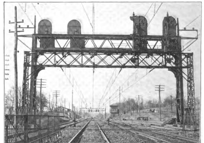
The Old and New Types of Signal Bridge on the Electrified Section.
