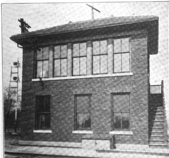
Concrete and Brick Interlocking Tower.
