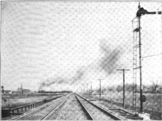
Home Signal 37 at Danger; Train on Wye Track.
