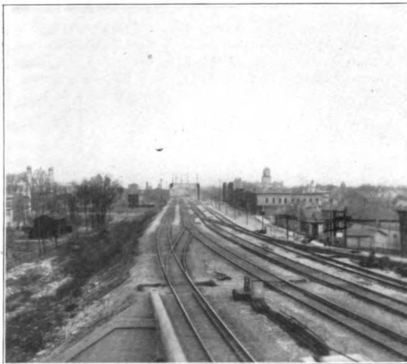
Fig. 5. View of Signal Bridge Looking North on the Rock Island and Michigan Central.
