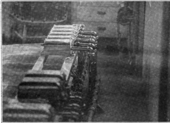
Fig. 8. Interior Wiring Construction, Using Conduits.
