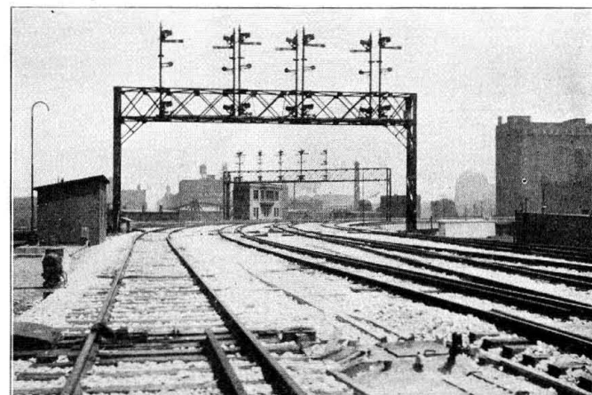
Fig. 5. Clinton Street Tower, Showing Signal Bridges.
