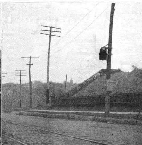
Fig. 3. Signal at the South End.
