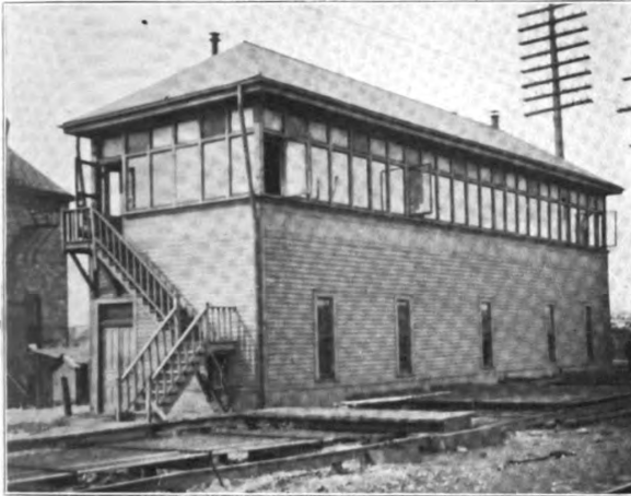
Fig. 1. Burnside Interlocking Tower.
