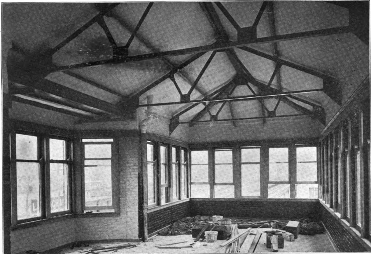
Second Floor of Tower—Showing Steel Construction.
