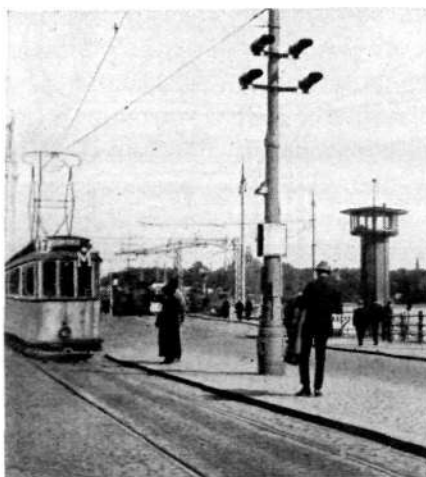
R 152. Fig. 2. Traffic Signal Mounted on Tramway Pole.
