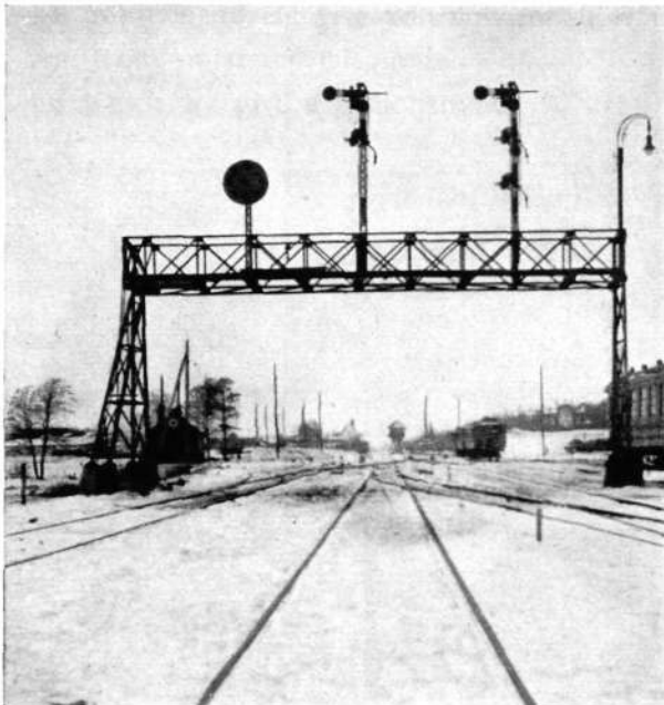
Signal Bridge in North Signal Cabin Zone.
