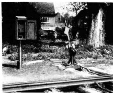
Fig. 4 X 5442 Key locked points with electric key central
