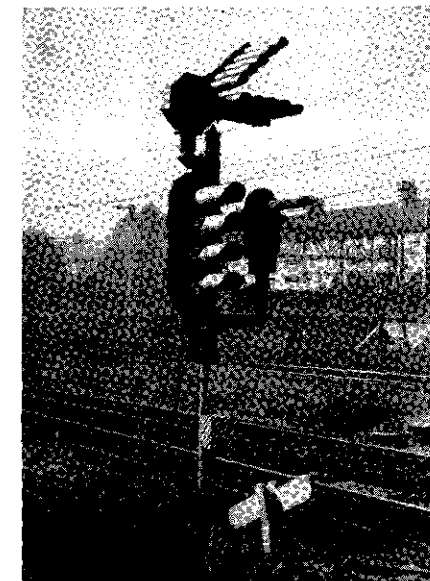
Fig. 12 Junction Indicator 5 Lamp Non-Pivot
