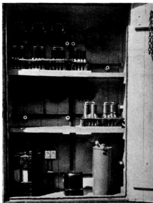
X 1279 Fig. 15. Relay cubicle at a block station along the track. Top and middle, relays and choke coils; below, storage battery with charging equipment.
