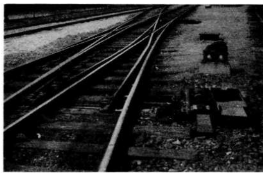
Fig. 21. Double crossing points, with double drive.
