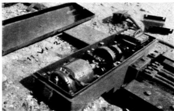
Electric Switching Machine.
