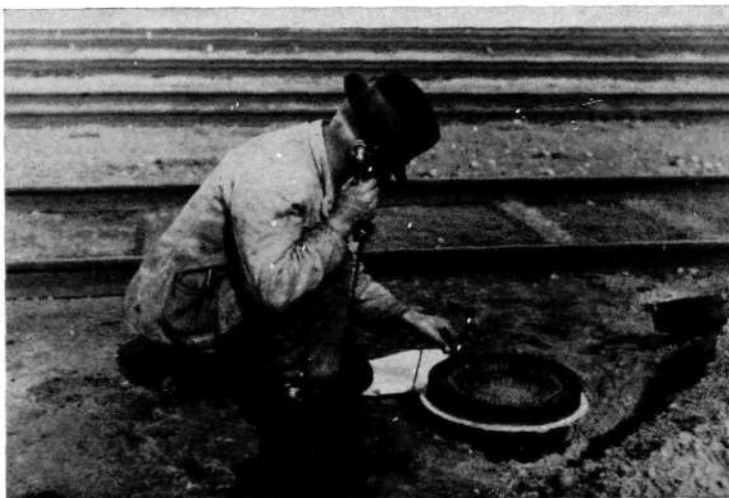
Fig. 25. Testing a cable distribution box.
