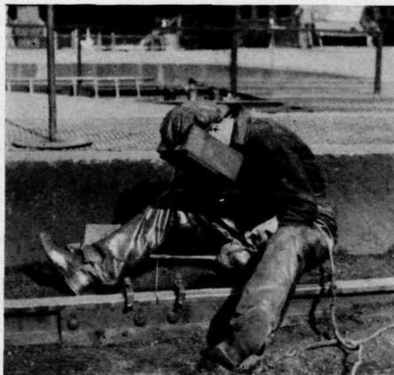
Fig. 23. Welding of rail bond.
