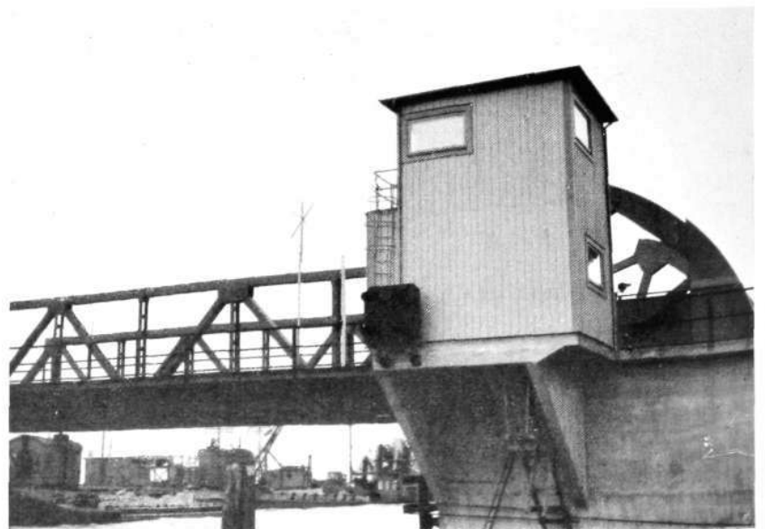
Fig. 3 X 5814 Control tower of the bascule bridge
