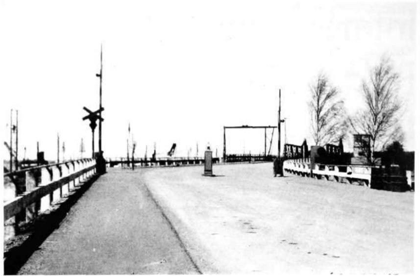
Fig. 2 X 5803 Lifting gates, illuminated signals and traffic dividers at the entrance to the bridge
