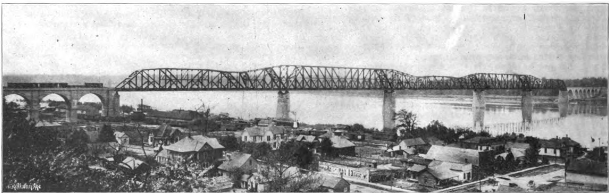
THE THEBES BRIDGE OVER THE MISSISSIPPI RIVER—GENERAL PLAN OF THE COMPLETED STRUCTURE.
