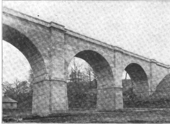
THEBES BRIDGE—ILLINOIS APPROACH.
