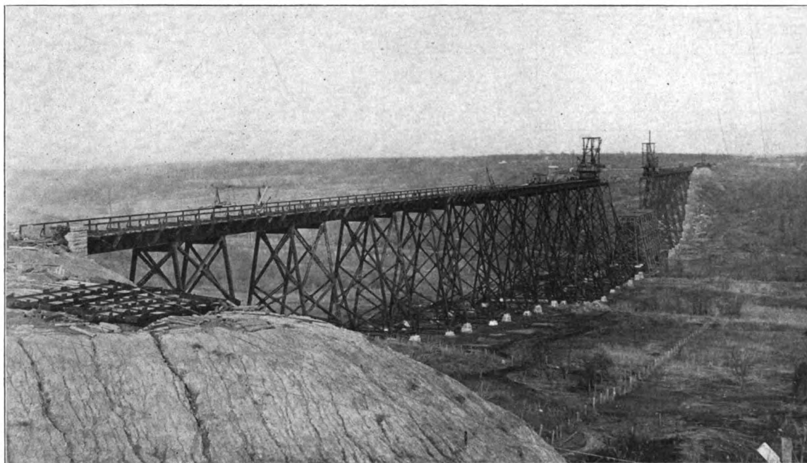
VIADUCT AT BOONE, IOWA, CHICAGO & NORTHWESTERN RAILWAY—SHOWING TRAVELERS AND FALSE WORK IN PLACE PREPARATORY TO ERECTING CHANNEL SPAN. From photograph taken March 18, 1901.
