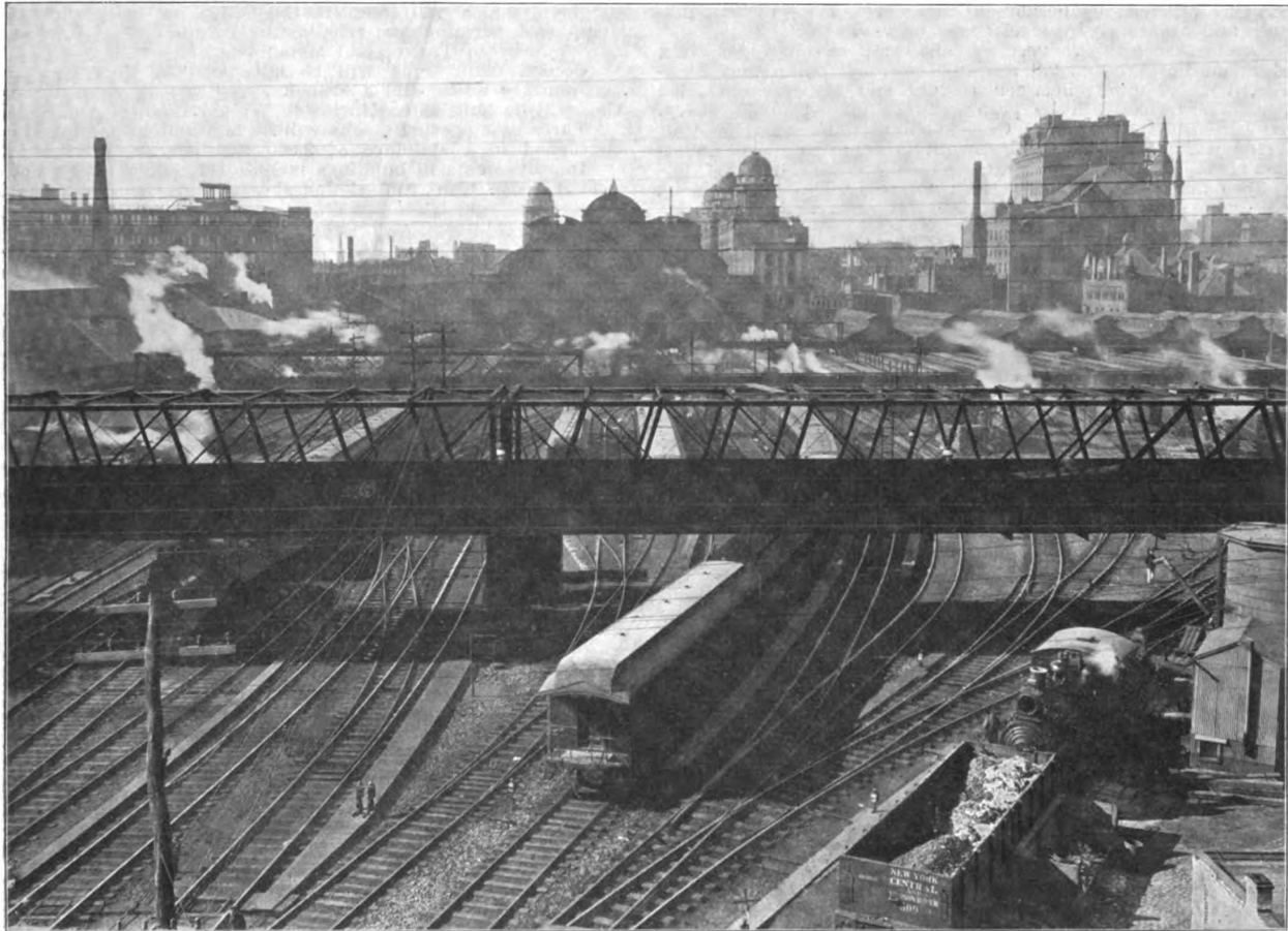
INTERLOCKING PLANT IN THE YARDS OF THE GRAND CENTRAL STATION, NEW YORK.
