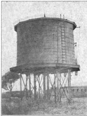
Fig. 3.—Water Tank Frame of Old Rails—N. & W. Ry.
