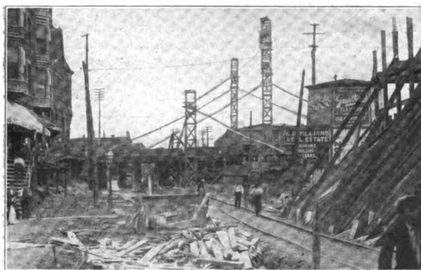
Looking East in Seventy-sixth Street During Work of Street Depression, Showing Distributing Towers for Placing Concrete Subway Abutments.
