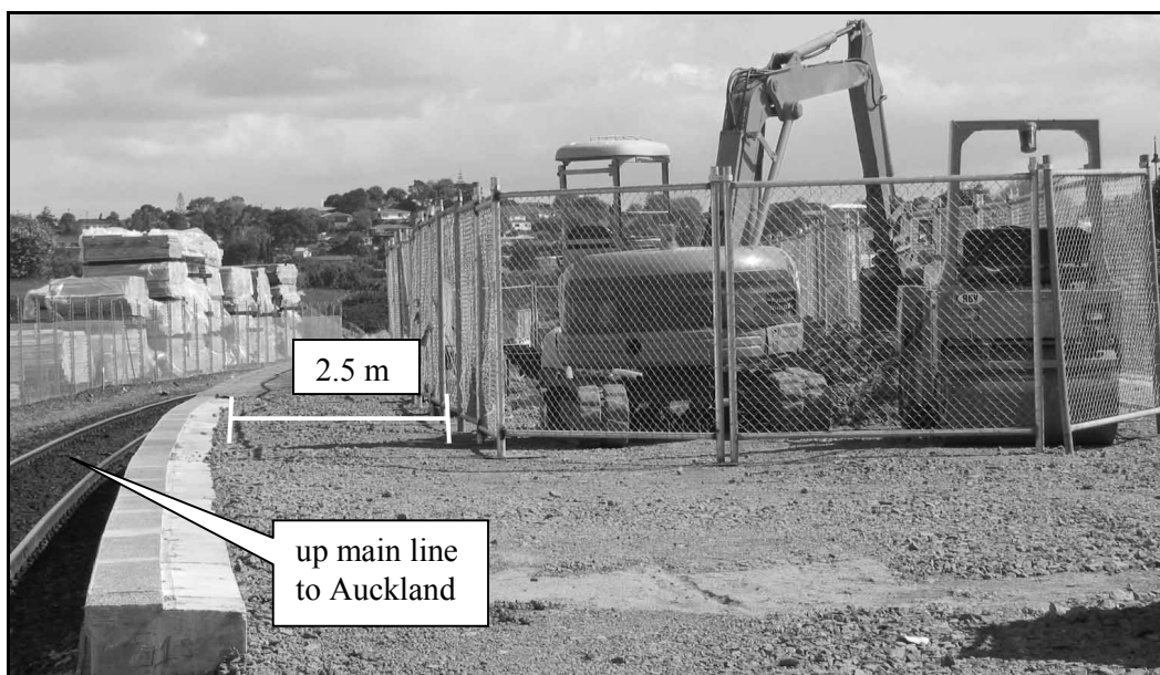
Figure 2 Construction work at Glen Innes Station
