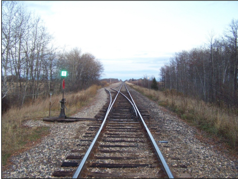
Photo 1. West switch at Meharry Siding looking eastward
