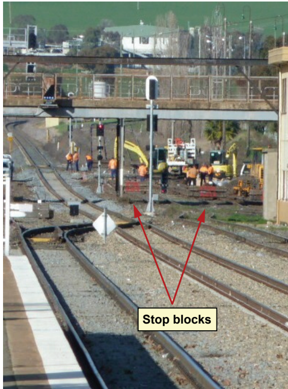
Figure 1: Worksite (looking south from Junee station platform) showing temporary stop blocks
