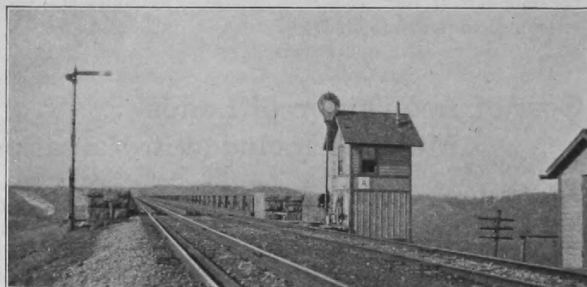
East End of Boone Bridge Showing Old Layout, Mechanical Home Signal Later Changed to Power Operated Signal
