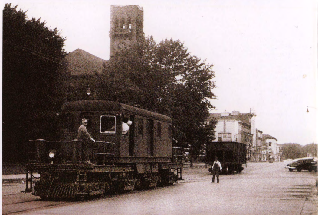
ABOVE: The east local is switching a car of coal for the Urbana power house, located north of the Champaign County court house. After the city street trackage through Champaign was abandoned, the Urbana trackage remained in place, permitting the "football specials" to access the Wright street team track located within the campus of the UoI. GEORGE ISAACS
